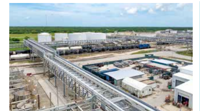
..... Glycol Railcar loading stations in Inland Traffic, TX
