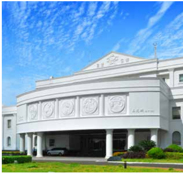
..... Administrative building in Mailiao Industrial Complex
