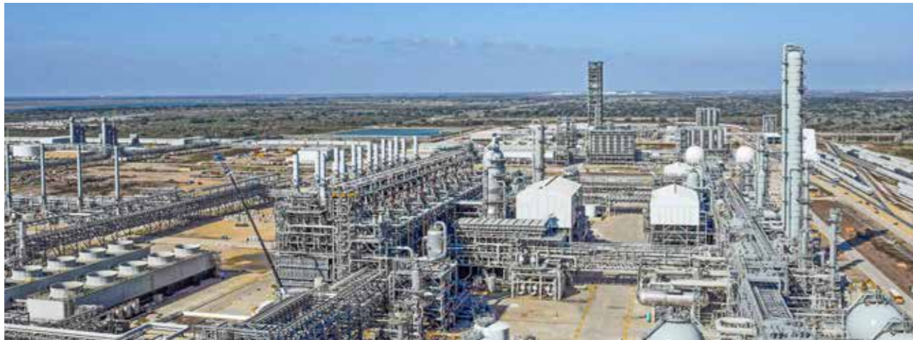
..... Olefins III Plant in Point Comfort, TX
